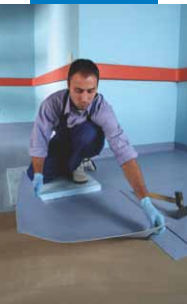
Installing PVC floor tiles
