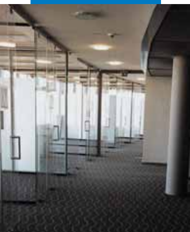
Carpet laid in Post Office Centre using Ultrabond Eco Fix - Post Tower - Italy
